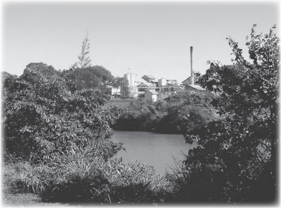
Looking across the Wilsons River at the Norco Lismore factory (present day).
