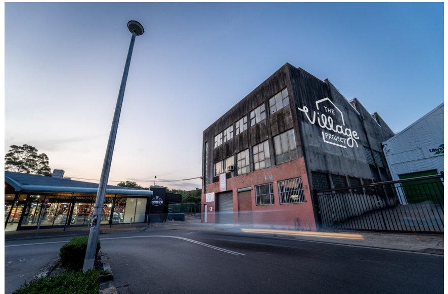
The Village Project Building Following images ©The Village Project
